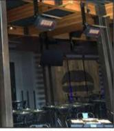
different areas, we have 4 switches which we can control zones where required." This feature allows restaurants to control their units with minimal effort and reduces the need for heaters to be on in an area not in use, saving the restaurant unnecessary gas costs.
